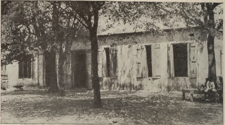
THE SCHOOL IN PORT AU PRINCE REBUILT BY MR. LLWYD
